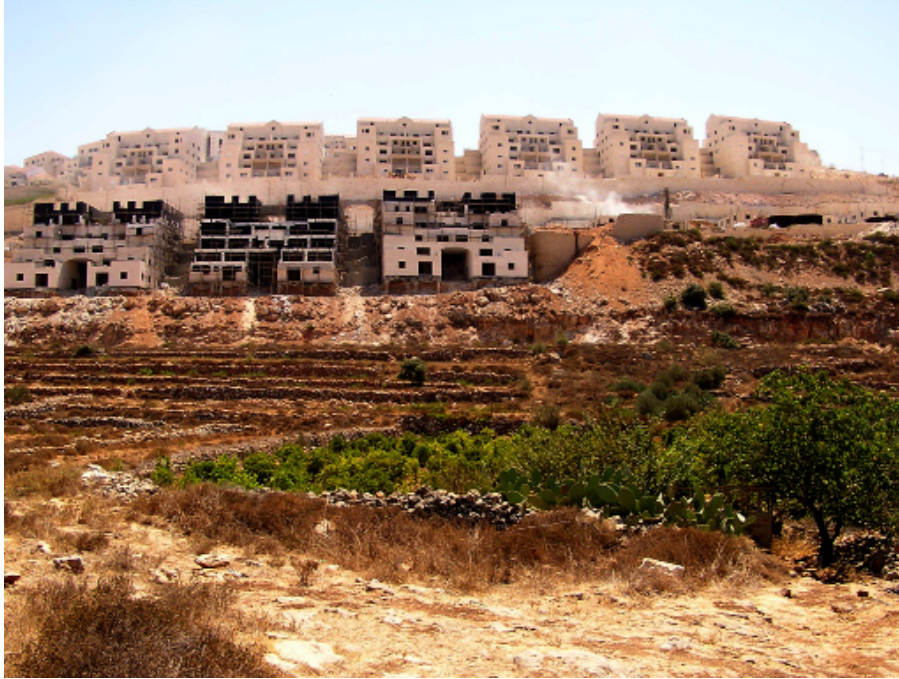
Figure 8 Beitar Eilit settlement construction encroaching on the land of Wadi Fukin
